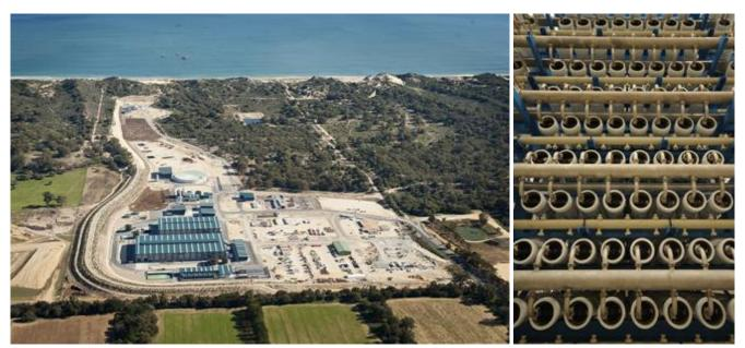
Southern Seawater Desalination Plant at Binningup WA and desalination membranes on site - Water Corporation
